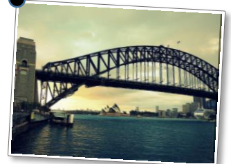
Sydney Harbour Bridge
