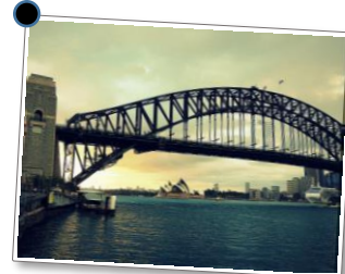
Sydney Harbour Bridge
